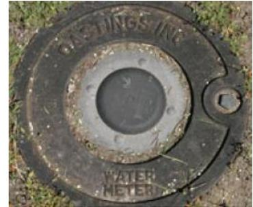
Meter pits are not designed to support the weight of a vehicle. Meter pits installed in driveways or parking areas often experience damage that can be very expensive to repair. In cases where meter pits are damaged in this manner the property owner will be responsible for repair or replacement.
