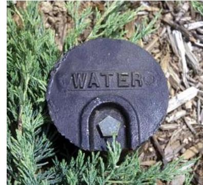
Over time, curb stop valves will wear out and become hard to operate, or the operating nut may break off. If the City of Durango Utilities crews are unable to operate the valve, they will repair or replace the curb stop valve as deemed necessary.
